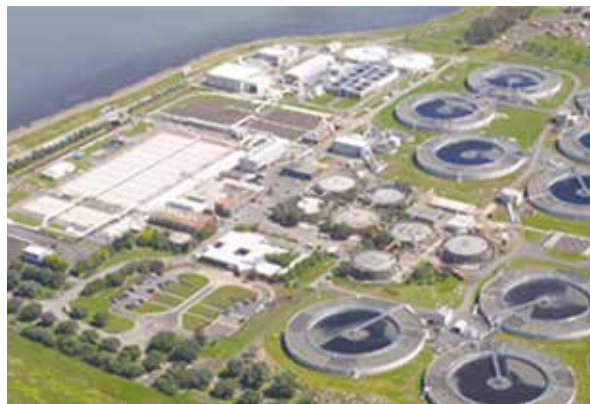
Figure 2. Municipal wastewater or sewage treatment plants (STPs) play an important role in removing pharmaceuticals, personal care products and other chemical contaminants from municipal wastewater
